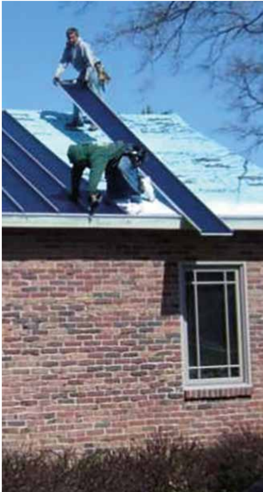
Roof integrated solar energy
