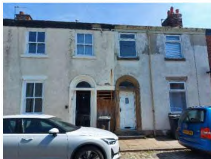
Painted brickwork; rendered elevation in poor condition
