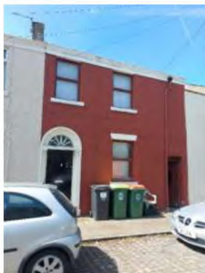
Painted brickwork; rendered elevation in poor condition
