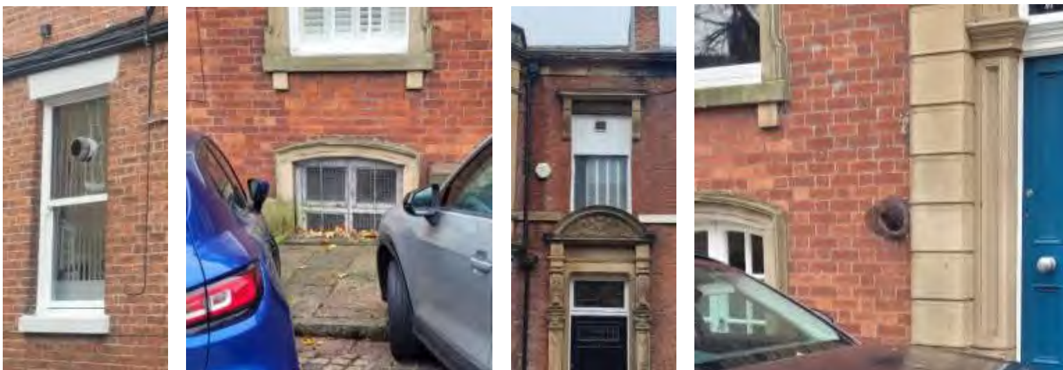
Vent in a window at Camden Place (left), security screen on window at Avenham Colonnade (centre left), altered window with vent at Ribblesdale Place (centre right), vent in wall at 5 Avenham Colonnade (right)
