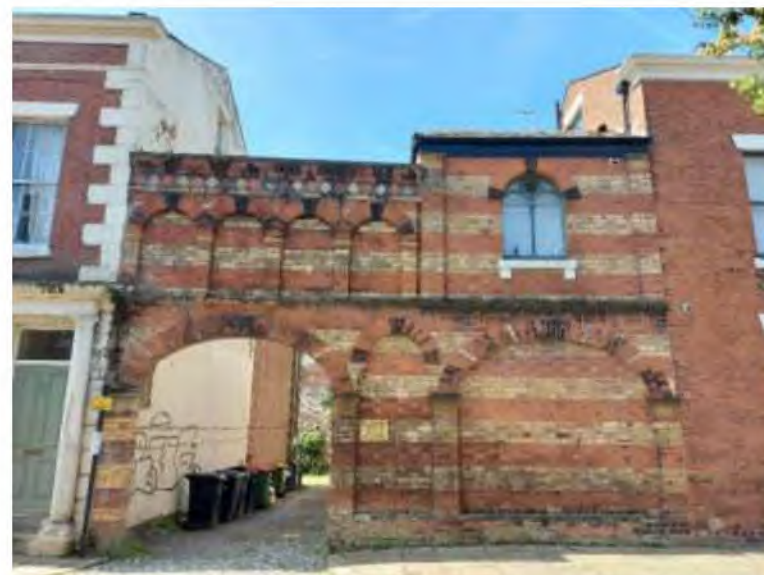
Polychrome brick wall on Latham Street and plastered quoins at either end of 22-28 Latham Street
