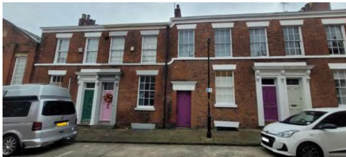
Traditional six over six timber sash windows on the northern end of Regent Street with door panels painted in a variety of colours
